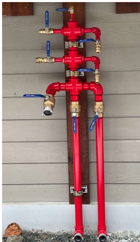
Primary manifold with ergonomic entry/exit to secondary manifold (not shown).
