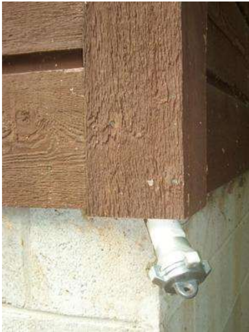
Concealed hard pipe sprinkler connection and permanent roof mount. These are excellent examples of permanent construction. Photo credit: onestopfire.com
