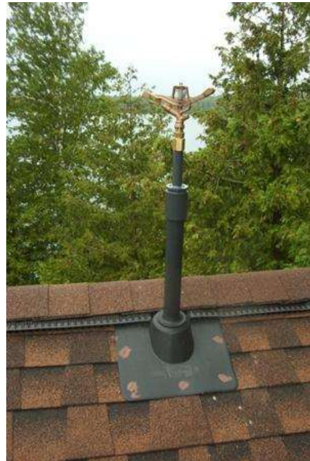
Concealed hard pipe sprinkler connection and permanent roof mount. These are excellent examples of permanent construction. Photo credit: onestopfire.com
